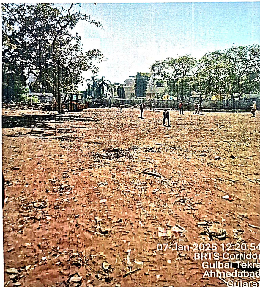
SITE PHOTO AS ON 07.01.2025
